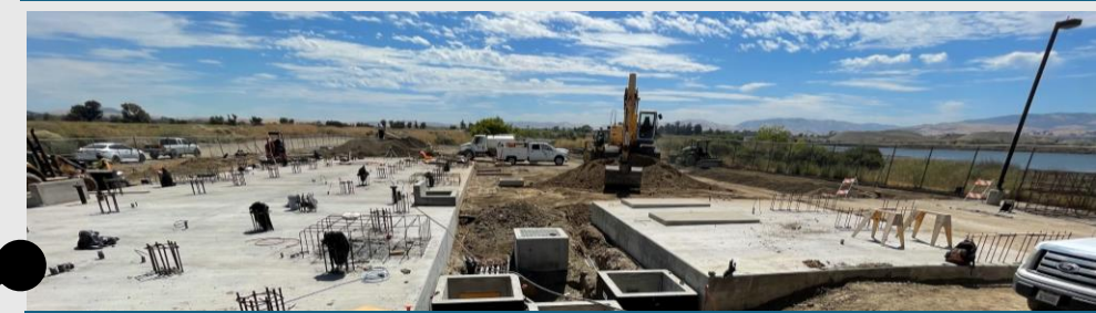
Chain of Lakes PFAS Treatment Plant Constructing Tank Pad, August 2024
