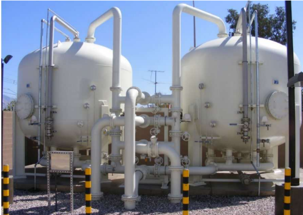
Figure 4 Example Pressure GAC Adsorption Lead-Lag Pressure Vessels
