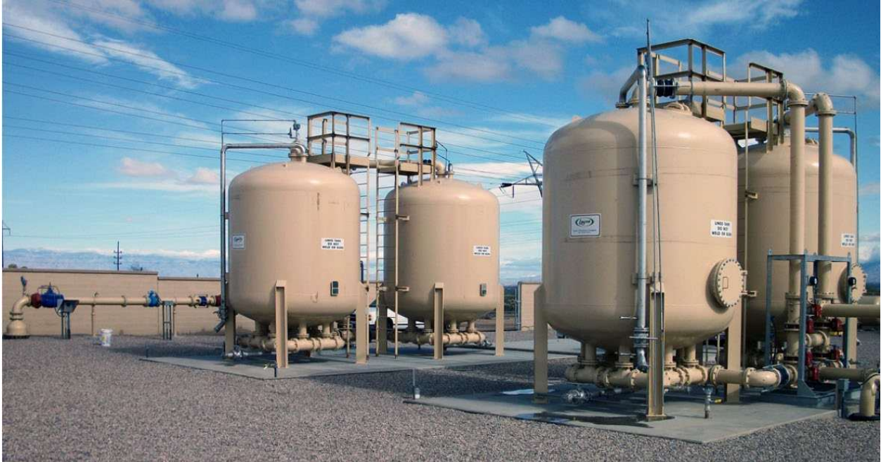
Figure 5 Example IX Pressure Vessels
