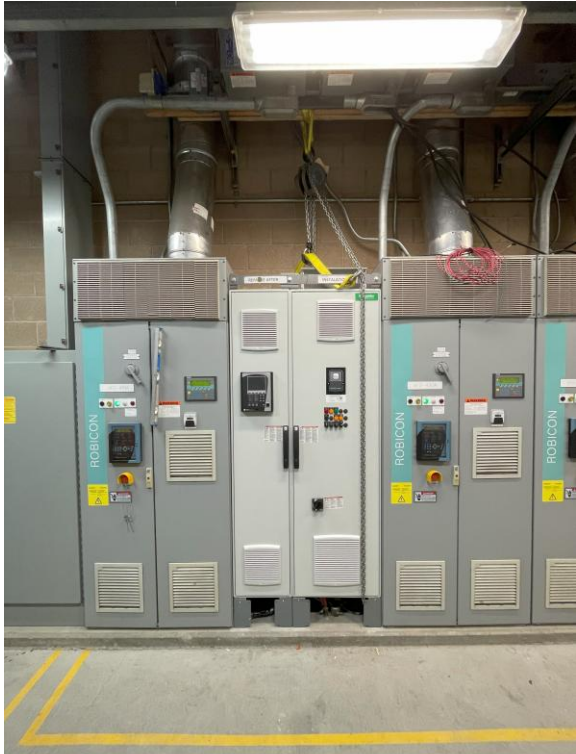
Wells & Electrical Upgrade/Replacement Project
