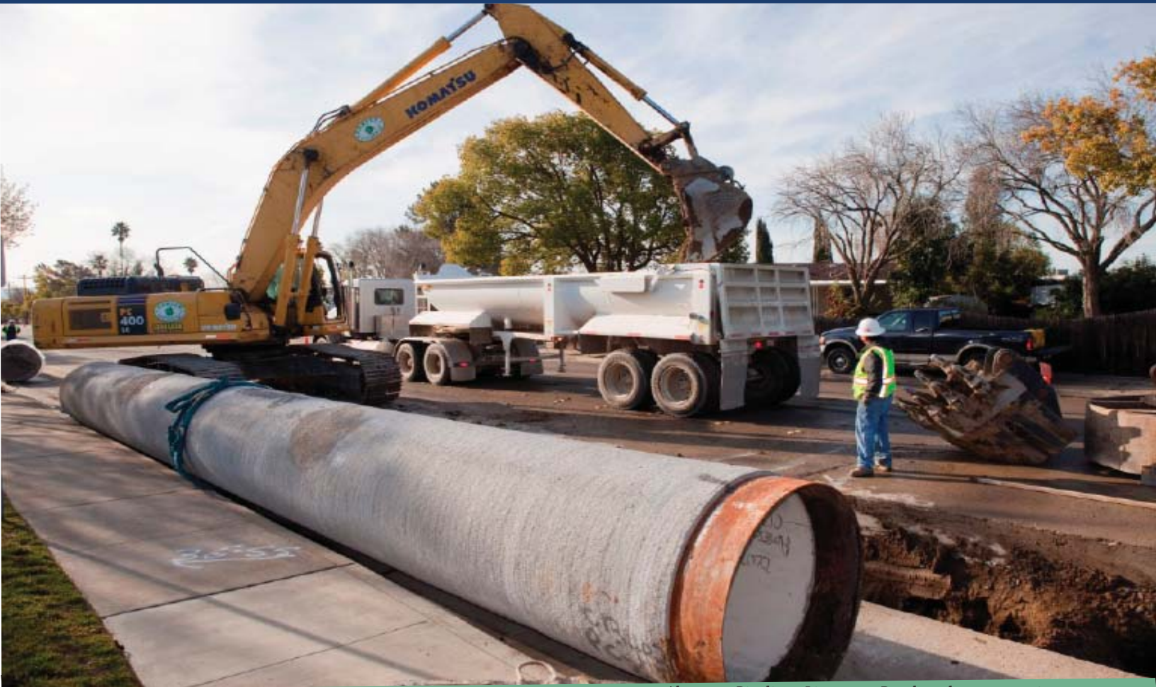
Altamont Pipeline - Livermore Reach under construction
