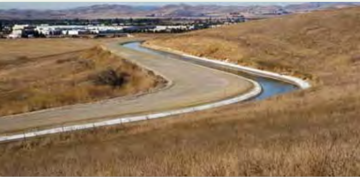
State Water Project's South Bay Aqueduct
