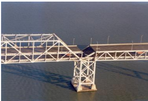
Collapsed San Francisco- Oakland Bay Bridge
