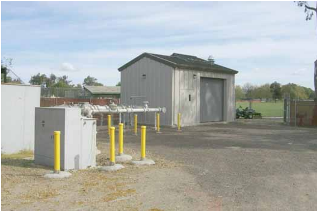
Building Type: Corrugated metal. Well Type: Well with Off-Site Treatment.
