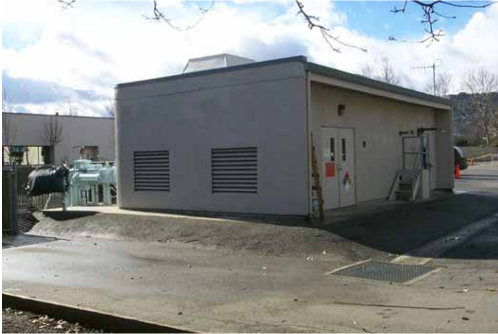
Building Type: Wood and stucco. Well Type: Well with On-Site Treatment.
