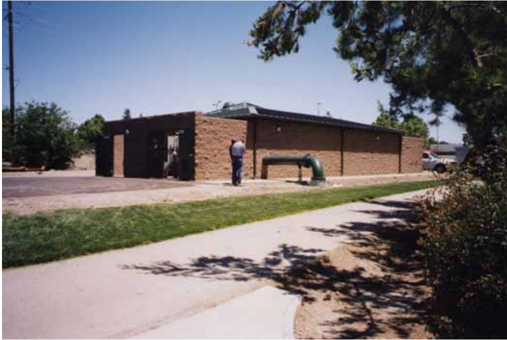
Building Type: Split faced cinder block and masonry block. Well Type: Well with On-Site Treatment.
