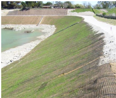
Recent slope repair at Cope Lake
