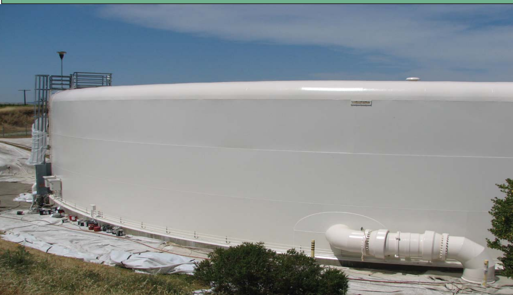
A Recently Recoated Clearwell at DVWTP
