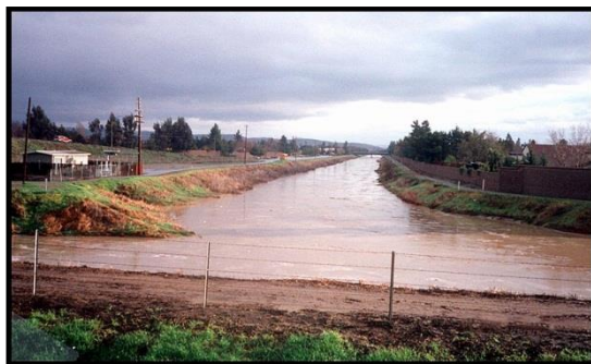
Existing Channel system providing flood protection after a large storm event in 1993
