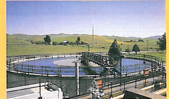
(Above) Clarifier at the 12-million-gallon-per-day Patterson Pass Water Treatment Plant. (Below) The 30-million-gallon Patterson Reservoir provides storage and helps equalize influent water quality to the Patterson Pass Water Treatment Plant.
